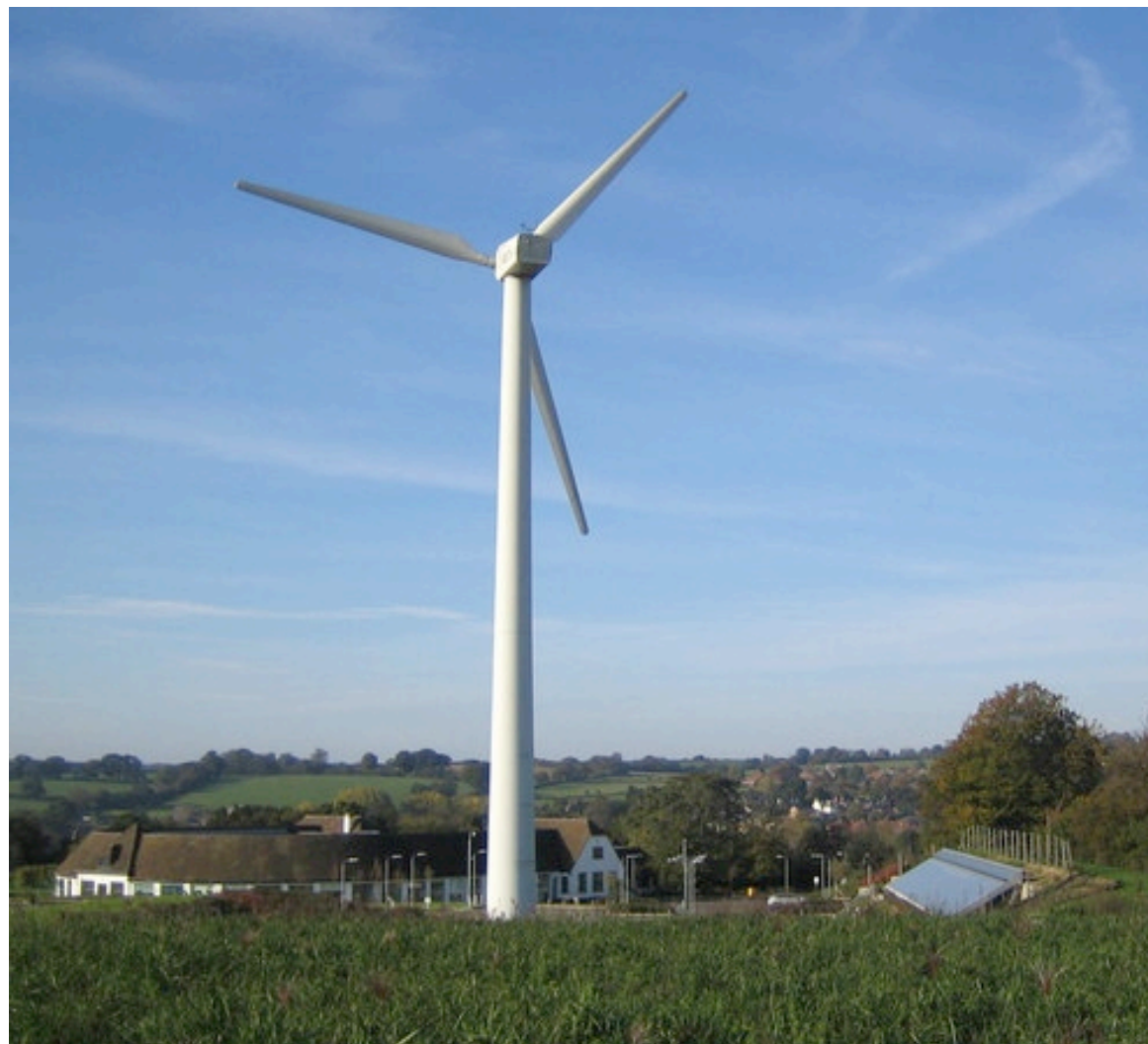
Kings Langley, 225 kW turbine
